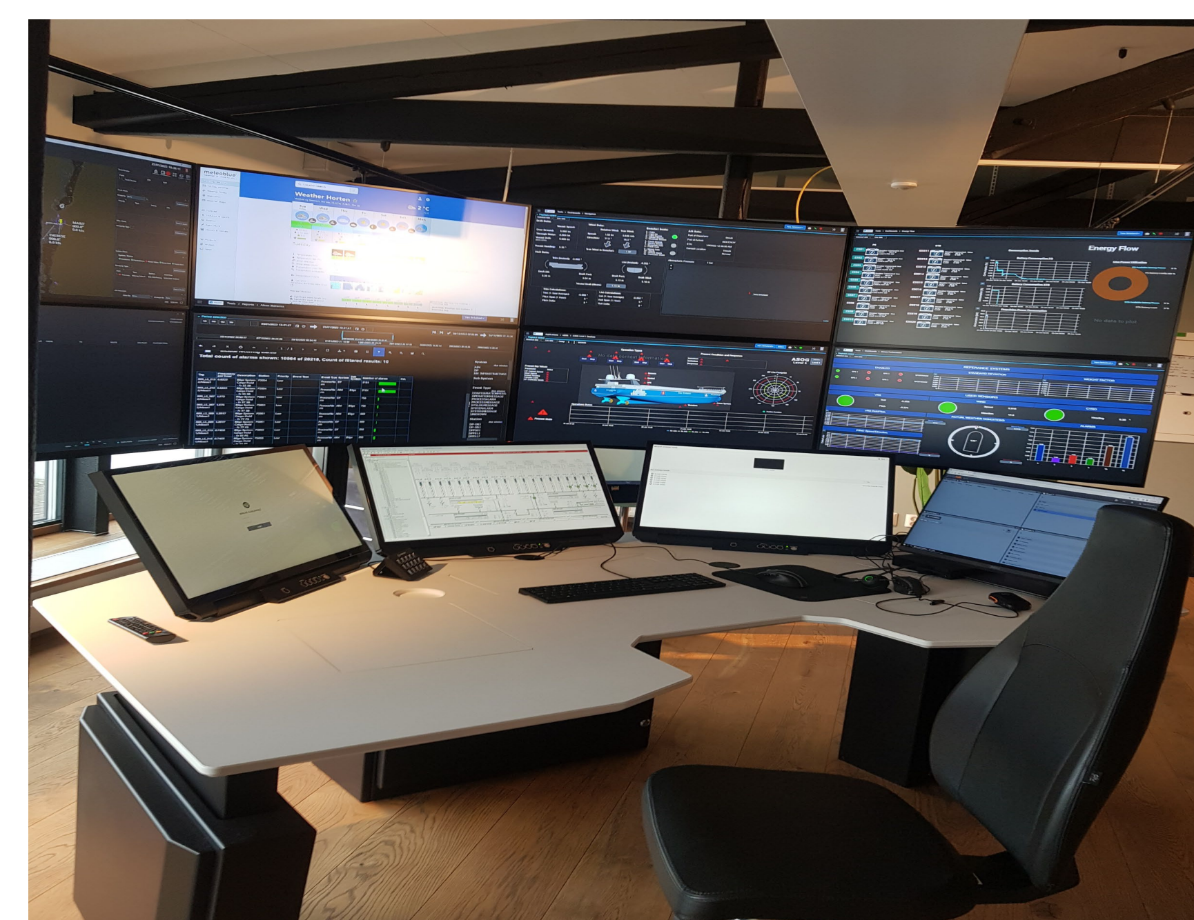
Figure-1: An example of Remote-Control Centre
