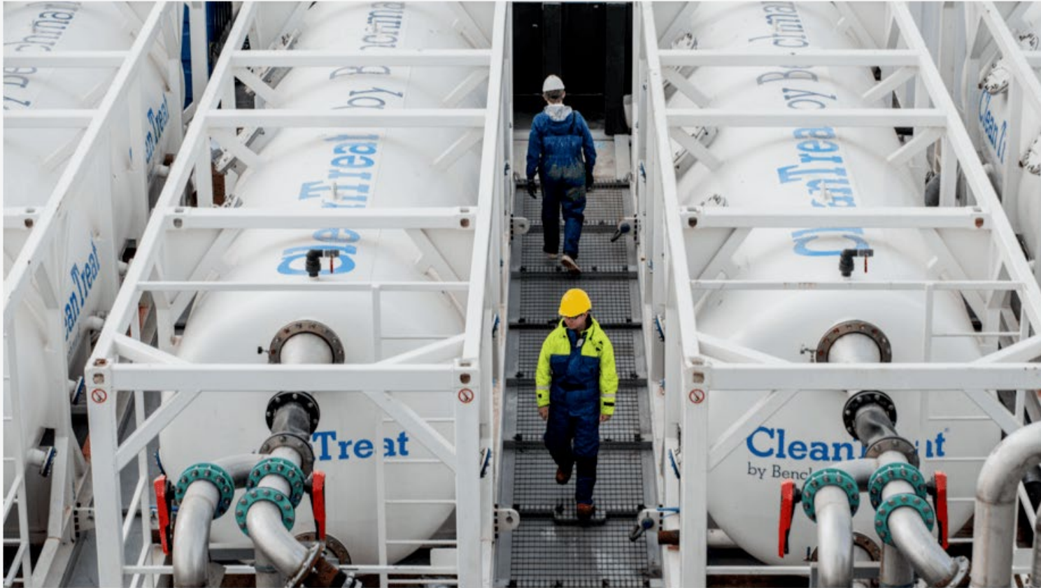
Benchmark's CleanTreat water filtration system enables BMK08 to be used without harm to the environment. Photo: Benchmark.
