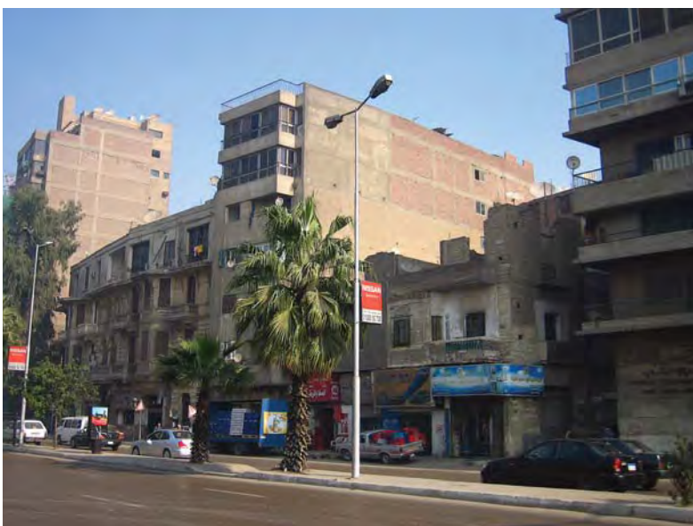
FIGURE 47. Buildings in poor condition along the Corniche in Old Cairo
