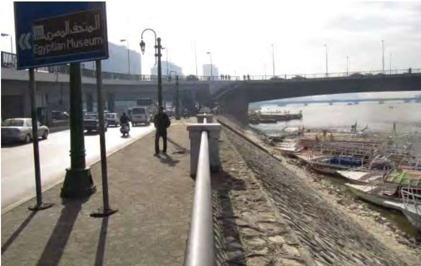
FIGURE 39. Concrete-lined levee along the Nile's east bank in CBD
