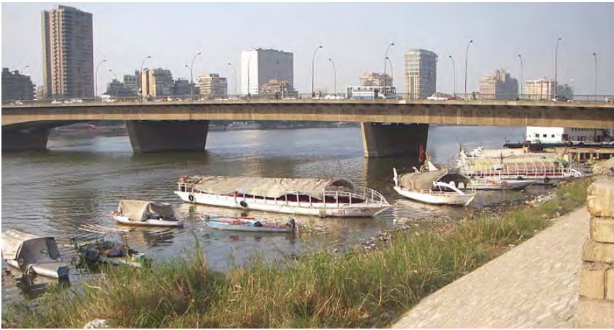
FIGURE 65. Steep concrete banks, unused terraces, and informal settlements along the water's edge
