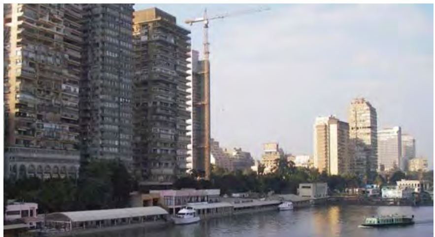
FIGURE 33. View of the Nile's west bank in CBD from the Al-Gamaa Bridge
