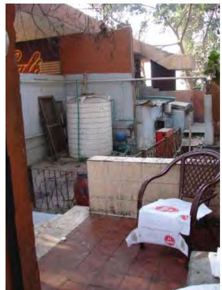
FIGURE 10. Blocked access Ventilation units and storage facilities for private clubs prevent pedestrian access to the Nile waterfront from the sidewalk.
