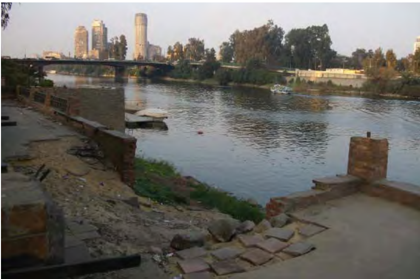
FIGURE 40. Unused lower terraces
