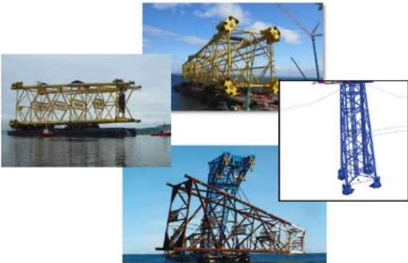
Figure 2-2: Typical 4- leg Jackets
